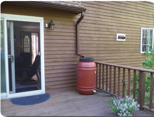
Rain barrel attached to gutter downspout.
