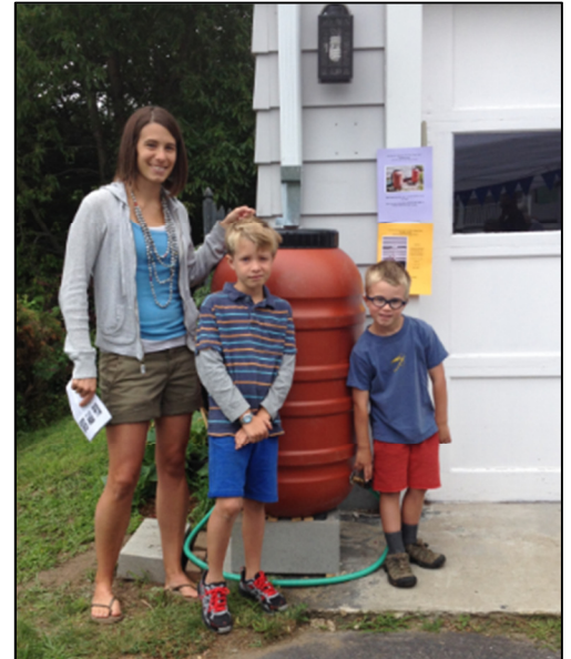
Neighbors check out a rain barrel installed by SOAK Great Bay at this Dover home.
