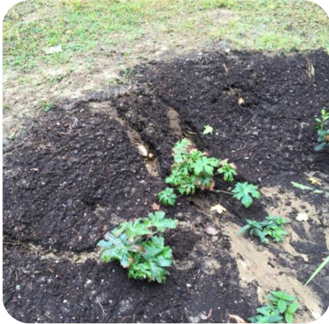
The upper bank experienced erosion during a large storm. Additional plantings on the bank helped address this issue.
