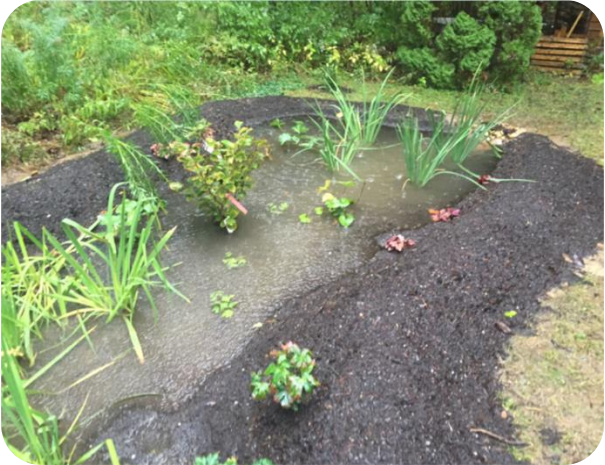
This Mill Pond Road neighborhood rain garden captures runoff from paved and grassed areas potentially reducing pollutants and excess flow to the Oyster River.
